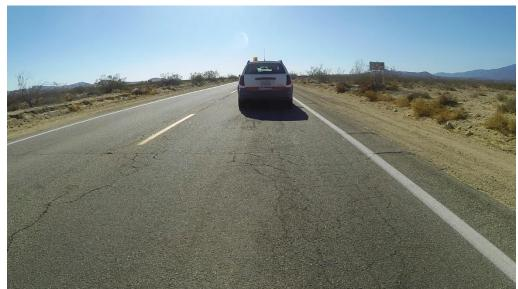
Distresses were reflective, block cracking and alligator cracking. There was located processorial of base failures which made this a great candidate for a CIR.
